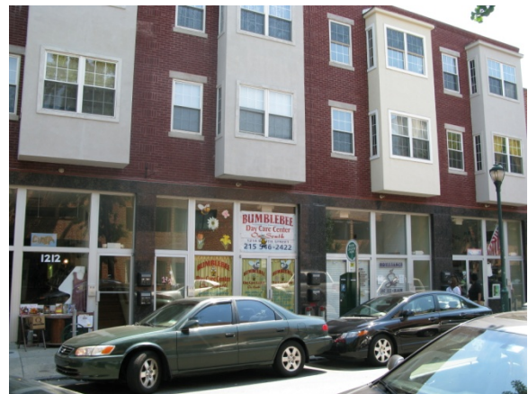
1212-1220 South Street; Multi-story mixed use development with ground floor retail. Photo Credit: Lynn Mandarano, 2012.
