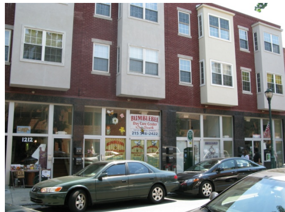
1212-1220 South Street; Multi-story mixed use development with ground floor retail. Photo Credit: Lynn Mandarano, 2012.
